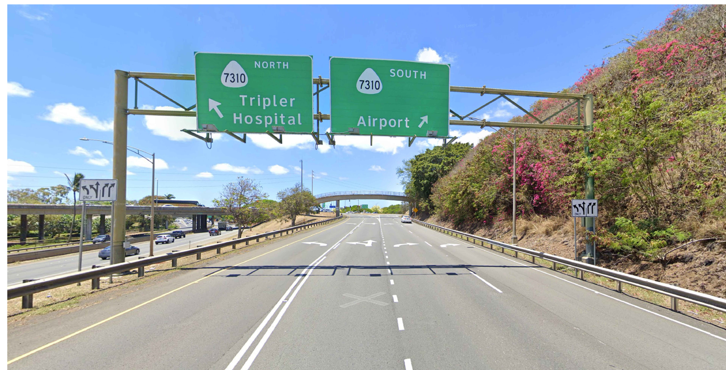
EXISTING SIGN STRUCTURE 78EBR-830
