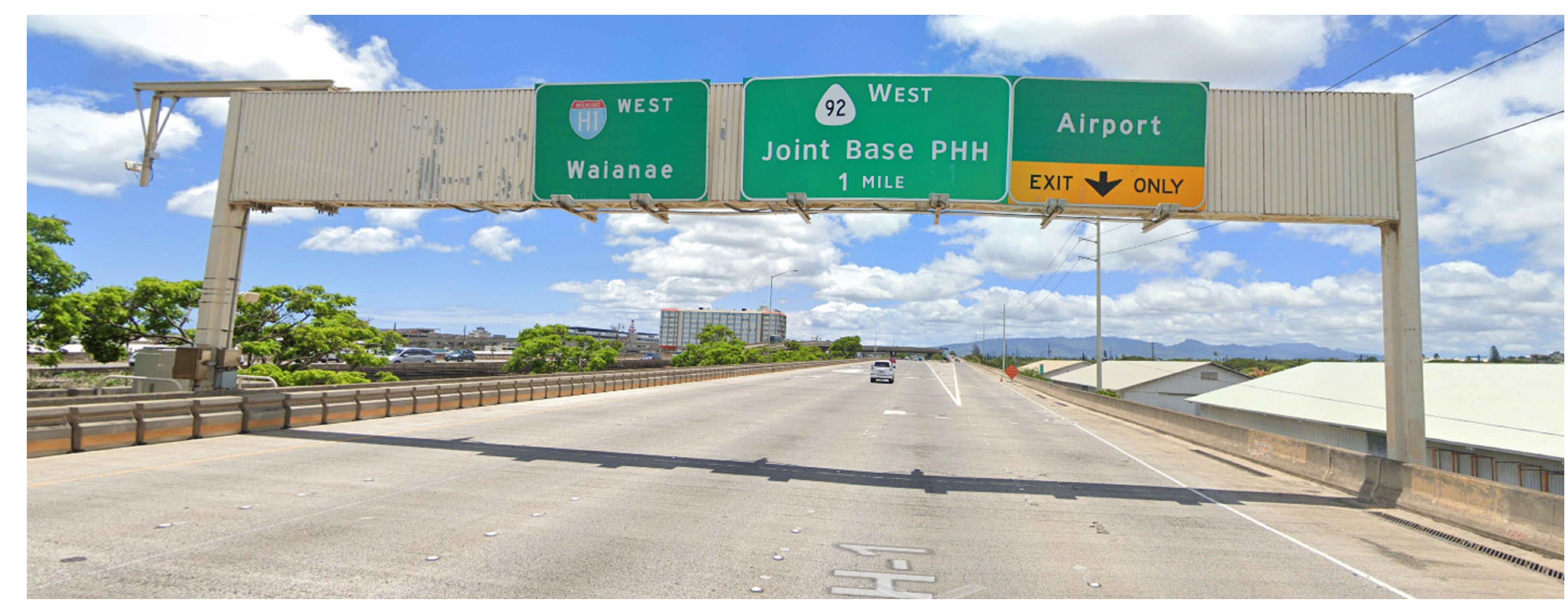
EXISTING SIGN STRUCTURE HIWB-505
