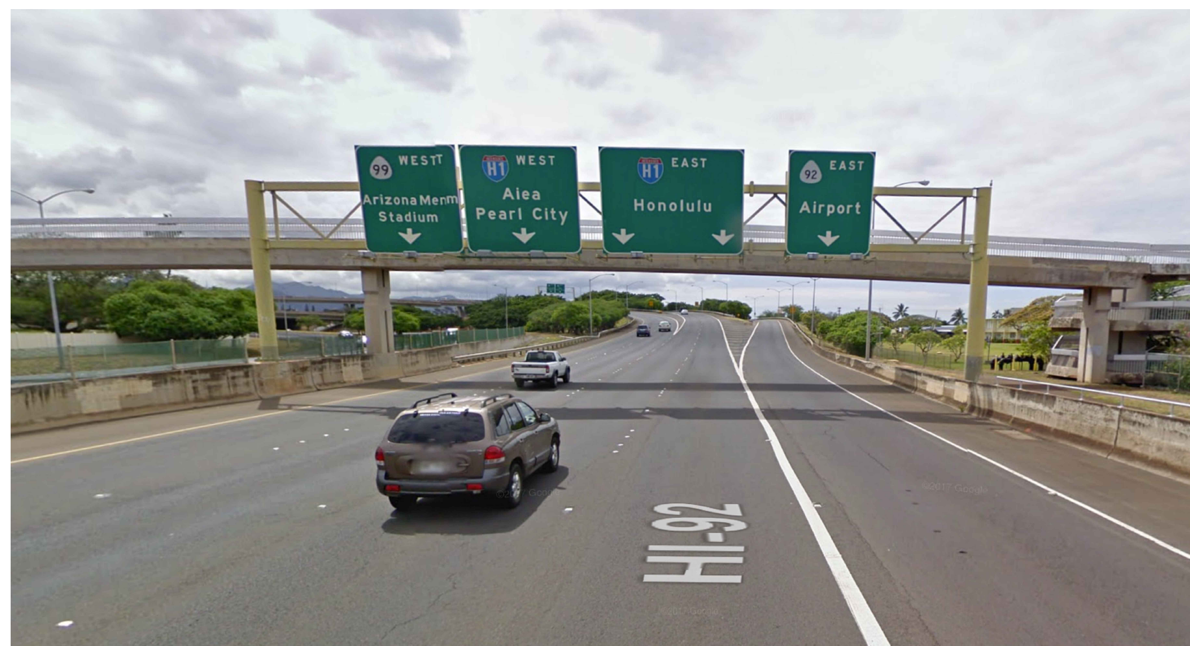
EXISTING SIGN STRUCTURE HIEBR-253
